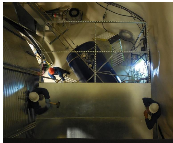
LN 2 -cooled storage dewar underground
